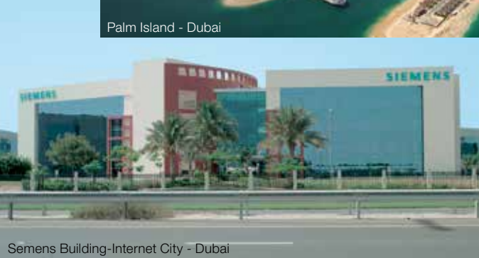
Semens Building-Internet City - Dubai
